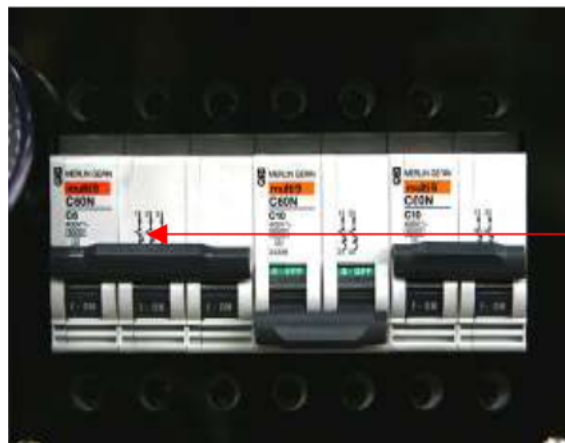
<Fig. 4-1 Main Power Switch>
